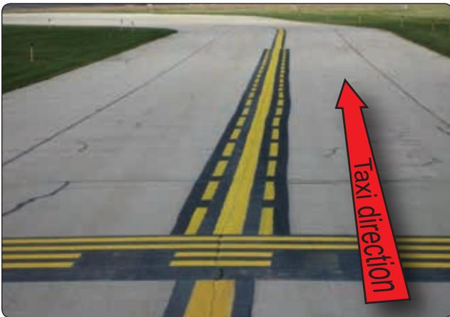
Figure 14-14. Runway holding position markings as seen when exiting the runway. When exiting the runway, no ATC clearance is required to cross.
