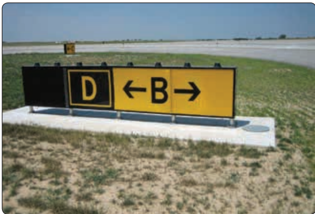
Figure 14-18. Taxiway Bravo direction sign with a collocated Taxiway Delta location sign. When the arrow on the direction sign indicates a turn, the sign is located prior to the intersection.
