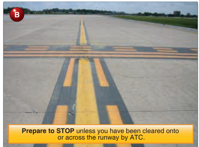
Figure 14-21. (A) Enhanced taxiway centerline marking. (B) Enhanced taxiway centerline marking and runway holding position marking.
