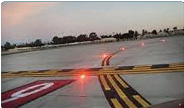
Figure 14-35. Runway Entrance Lights (REL).
