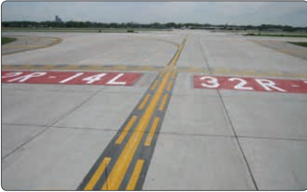
Figure 14-12. Surface painted runway holding position signs for Runway 32R-14L along with the enhanced taxiway centerline marking.
